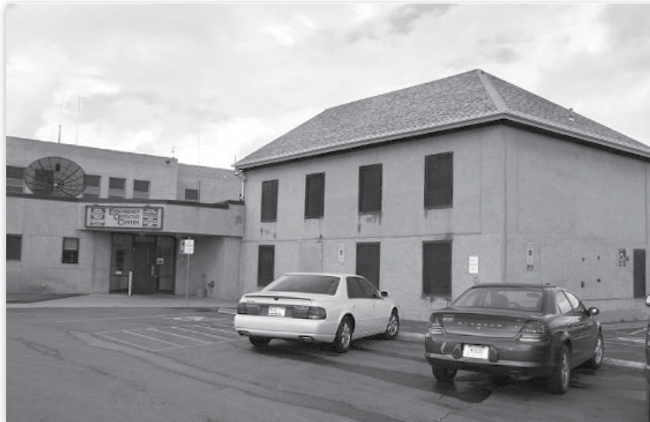
Custer County Detention Center
